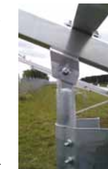
Juwi's mountings are three metres long and include up to ten kilos of aluminium components.
